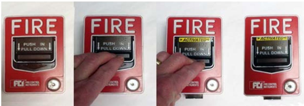
This newer style fire alarm pull station requires that you push in and then pull down. Please note - the **“Activated”** sign will appear when the device has been triggered.
