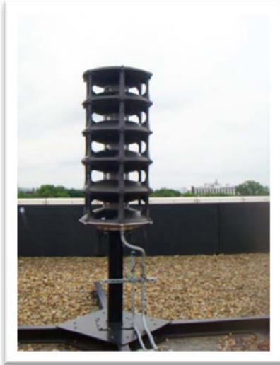
Brown University has installed an outdoor emergency siren system on its main campus. The system consists of three (3) strategically placed sirens that will be used to warn the University community in the event of a life threatening emergency with no advanced warning.
